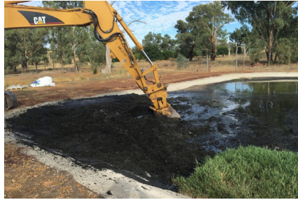
Mixing reagent on site
